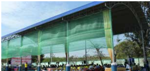
Steel Dome Project in Thailand
