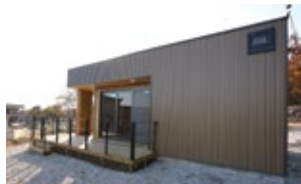
↑ Steel House built with POSCO corrugated steel plates for fire-stricken family
