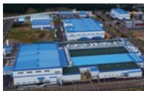
↑ POSCO Energy's fuel cell plant in Pohang
