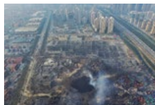
↑ Disaster at Tianjin Port
