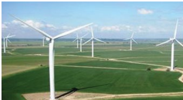
↑ Wind power generation
